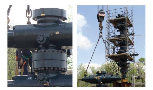
A large North American midstream company operating a gas storage facility required connection integrity management for a planned casing reroute. Due to damaged casing as a result of salt fall within the cavern, the said operator required a large Snubbing stack installation to handle the cavern pressure and capable of cutting 10 3/4" casing.
